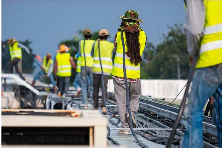
Figure 5: Workers Carrying Cable on Shoulders
